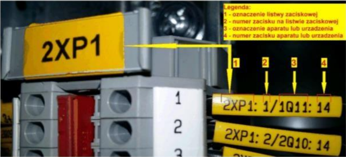
Photo. 7. Example of addressing wires on a marker
