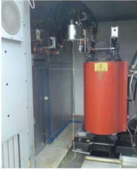
Photo. 8. Fastening of capacitor to non-load running compensator
