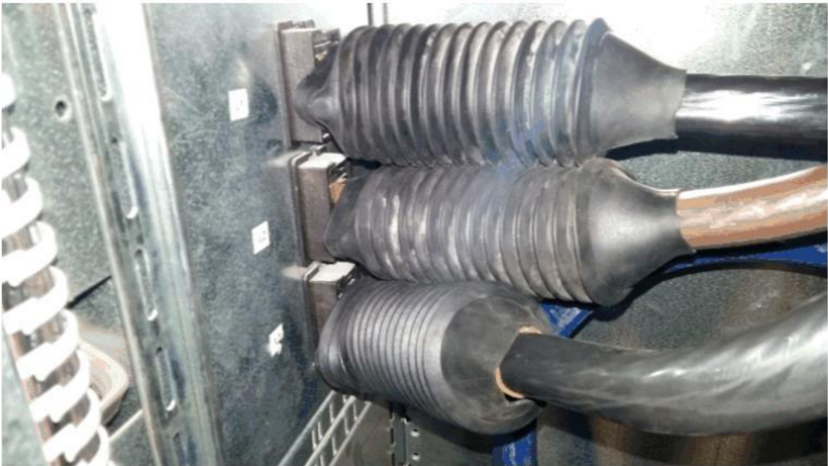
Photo. 2. Method of bellow assembly.
