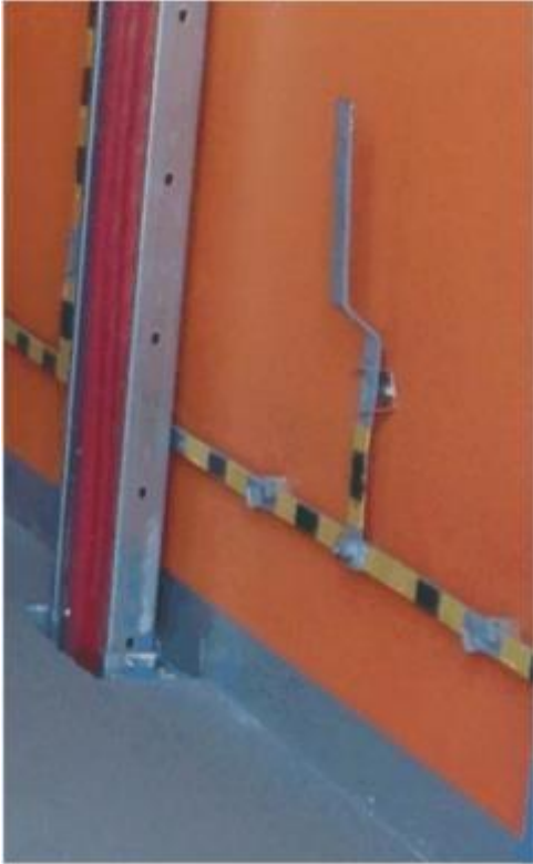
Photo. 12. A method for leading flat strip to the earthing terminal on portable earthing devices.
